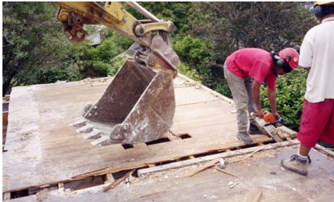
Salvaging wooden flooring (Ward Demolition)
