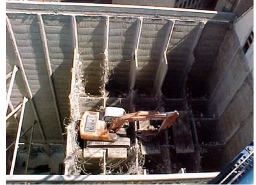
Deconstructing the Northern Roller Mill Building, Auckland (Ward Demolition)
